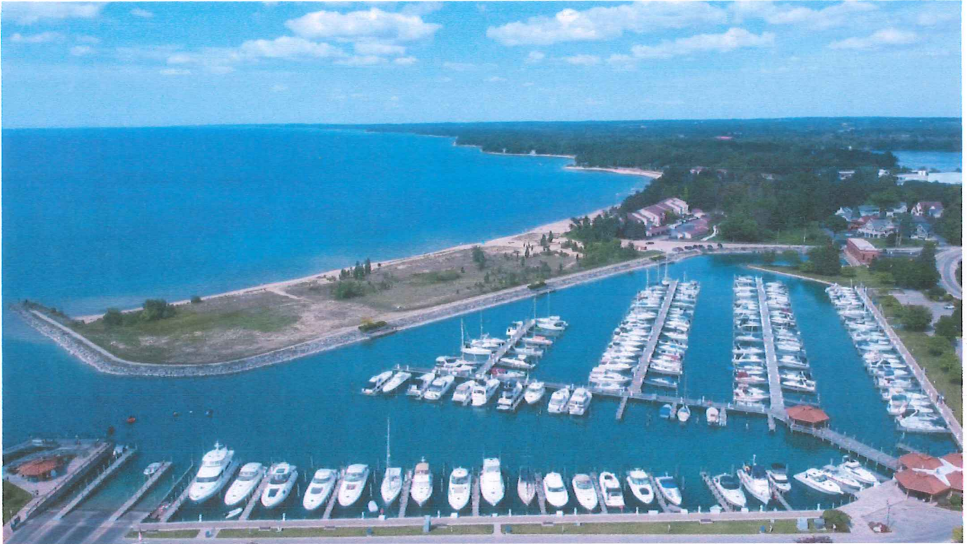
Figure 1: Aerial view of the Edward C. Grace Lower Harbor.
