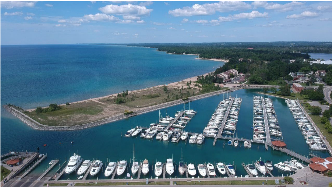
Figure 1: Aerial view of the Edward C. Grace Lower Harbor.
