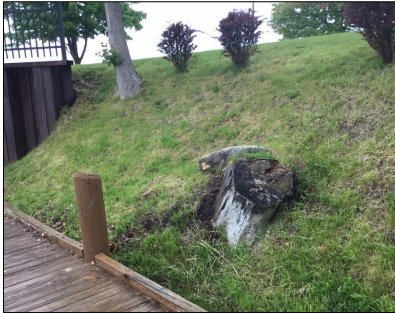
Points 2a and 2b have steep banks with high potential for future failures due to the poor stabilizing abilities of turfgrass
