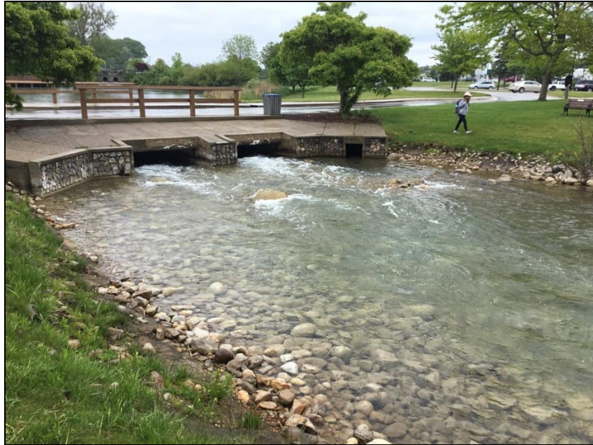
Point 2d: Minor erosion and bare soil along the bank on the west side of the Cedar Street bridge
