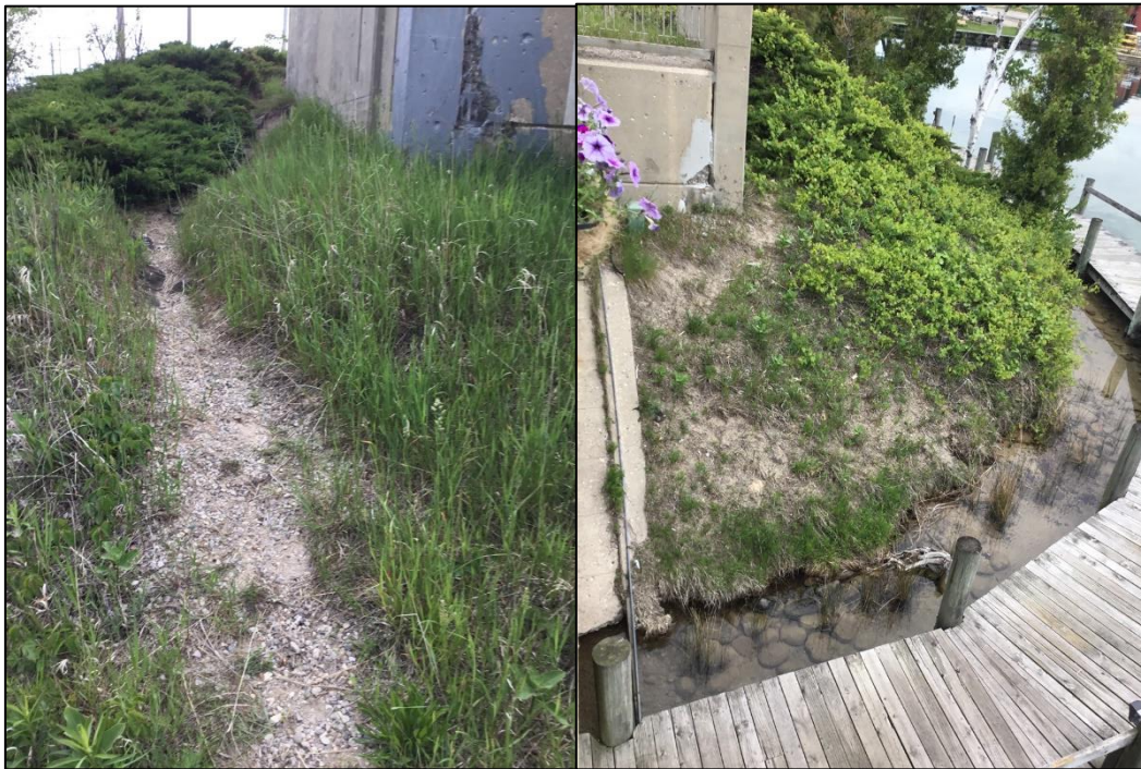
Figure 7: Points 4b (left) and 4a (right), showing bare soil and eroding path.
